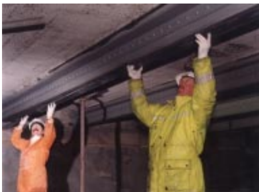
Figures 4 & 5: installation and temporary clamping of steel beams on Slattocks Bridge
