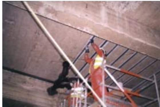
Figure 6: Strengthening floor slabs with CFRP plates
