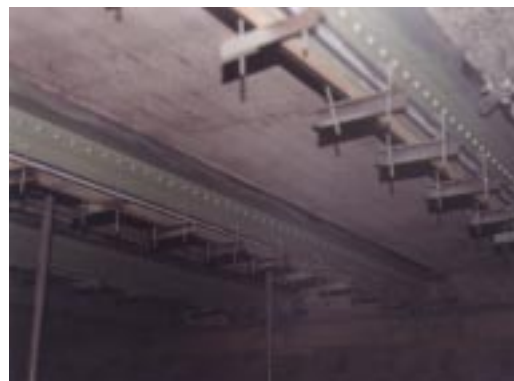
Figures 4 & 5: installation and temporary clamping of steel beams on Slattocks Bridge
